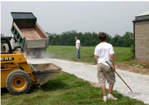
*Dave Houggy (in dump truck) spreads first layer of limestone in newly extended driveway.*
